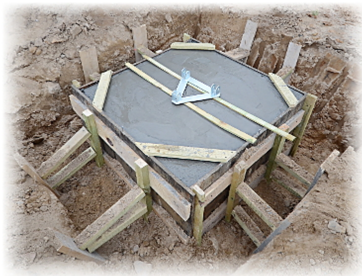
Ready foundation with the set mast:
